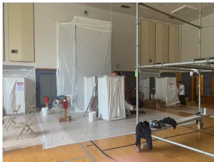
Before remodeling could begin, asbestos containment and abatement was required.
