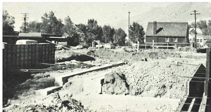
Footings and foundation are underway as the building is shown in early stages of construction.
